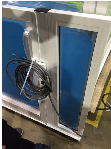
Figure 14 Attach filler panel to door/gate
